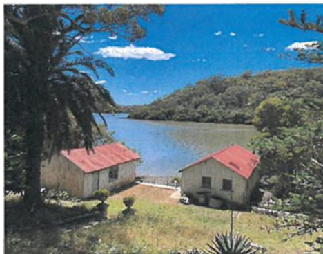
Figure 5.20 Showing the location of 45-6-1713, across the flat and artificially formed landform on which the boat sheds have been constructed. On the water's edge the landform has a sandstone retaining wall, beyond which mangroves grow. The wall has been infilled to a depth of 0.5m above the waterline. This landform would be entirely underwater with a 2m sea level rise.
