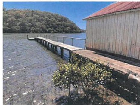
Figure 4.50 The jetty, adjoining the southern boatshed.
