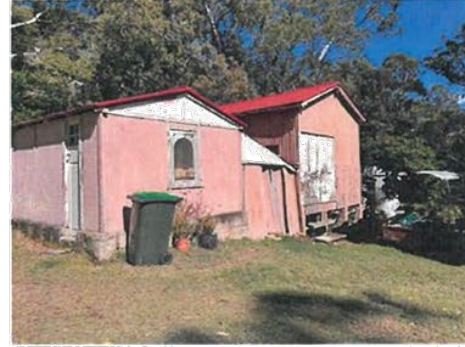
Figure 4.38 The garages, as viewed from the east.
