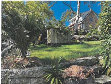
Figure 4.41 Cable-pulley engine shed.
