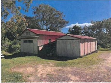
Figure 4.37 The garages, as viewed from the west.
