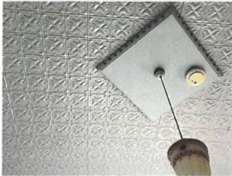
Figure 4.33 Pressed metal ceiling treatment in all three bedrooms.
